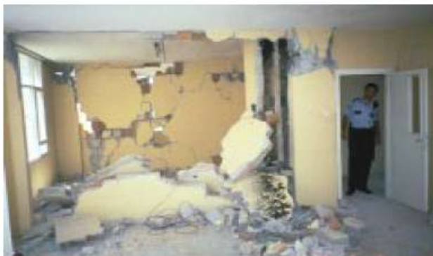
Figure 2 – Damaged columns as a result of increased lateral loads due to infill walls.
