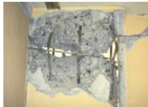
Figure 2 – Damaged columns as a result of increased lateral loads due to infill walls.
