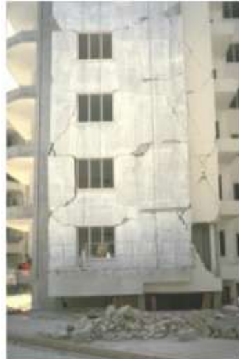
Figure 1 – A typical damage pattern due to lateral loads on a non-engineered infill walls.
